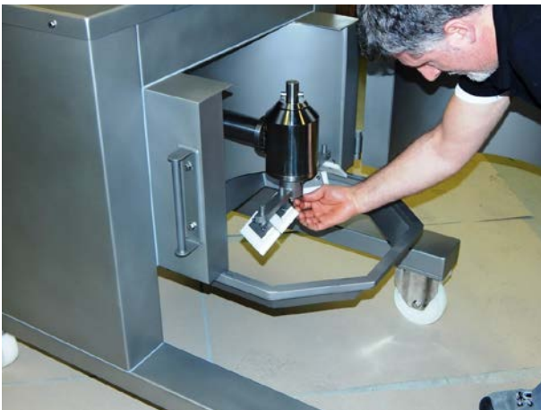
Fig. 13: Installing the scraper unit
